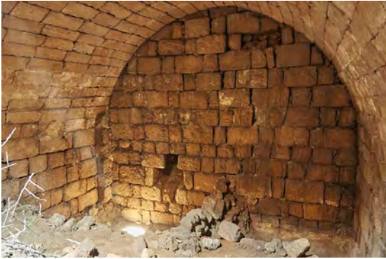
Fig. 1.95 East wall of cistern (Source: BAI/GPIA).
