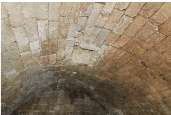
Fig. 1.99 Inner inlet of cistern (Source: BAI/GPIA).
